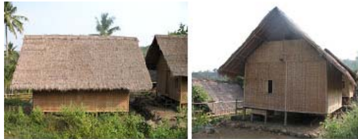
Figure 8: Overhanging roof of vernacular housing in Dukuh Kampong
