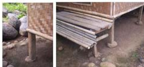
Figure 10: Stone foundation in Dukuh Kampong
