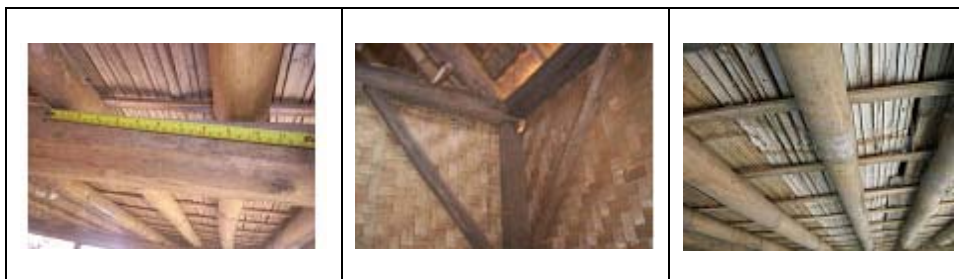
Figure 4: Connection and joint system in vernacular housing of Dukuh Kampong
