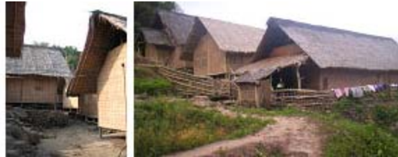
Figure 1: Raised box frame on vernacular housing in Dukuh Kampong
