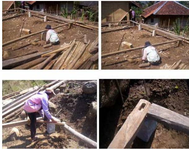
Figure 9: Local peoples construct their house
